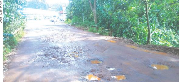
Potholes and loose gravel mar the road leading to Ponda's KTC bus stand
